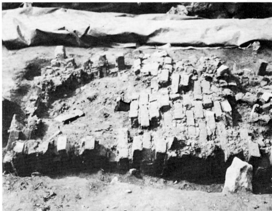
Fig. 5— Upper portion of fallen chimney at One Story Barracks, Fort Montgomery. —Palisades Interstate Park Commission photo.
