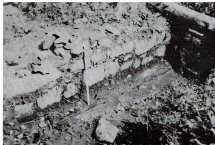
FIGURE 4. South race-way of Middle Forge with stone-lined side walls and remains of oak beams in the bottom.
