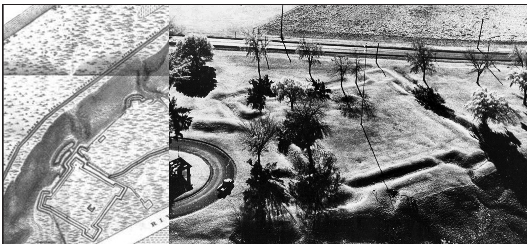
Figure 5. Smaller, second fortification at Meigs, photo taken in 1967 prior to removal of earthen fortifications (Nass 1980).
