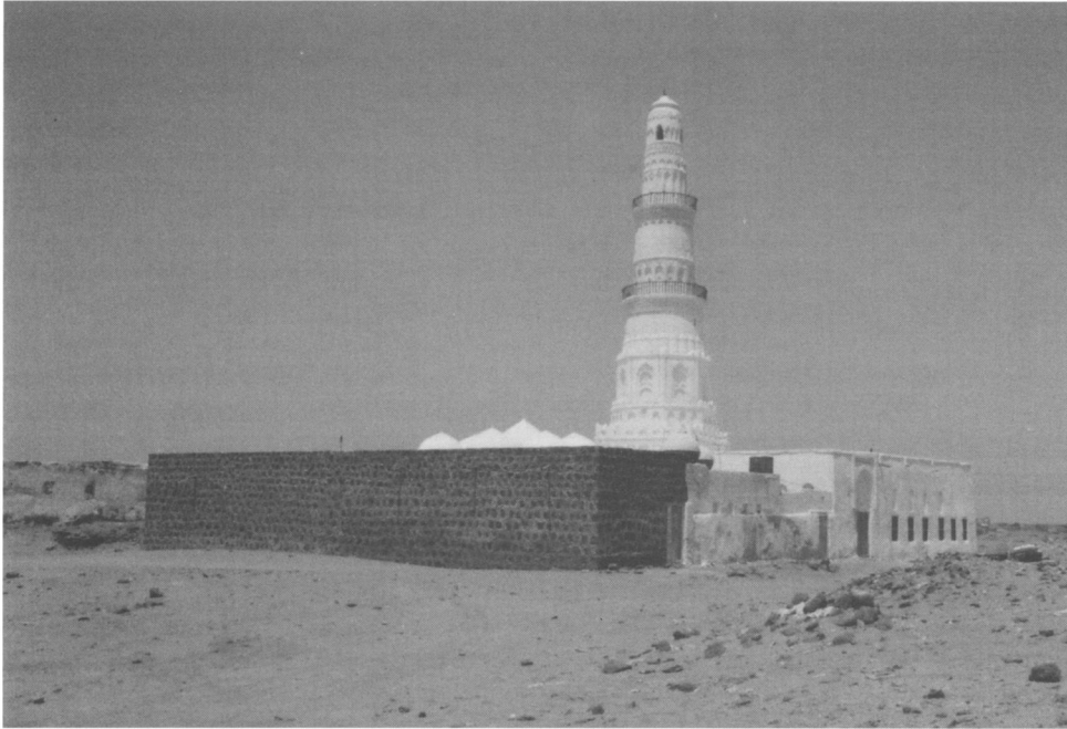
Figure 10 Mosque of al-Shadhili, Mocha, fifteenth century. The photograph shows the modern expansion in stone to the west of the historic mosque.
