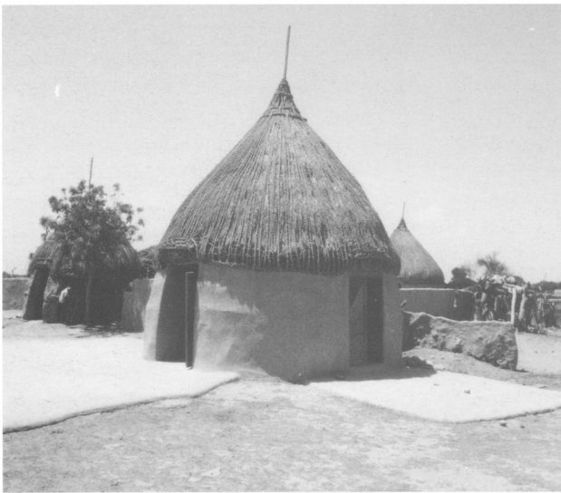
Figure 6 A reed-and-mud house in the village of al-Risas, Yemen. This type used to be dominant in the southern Red Sea coastal plain of Yemen.
