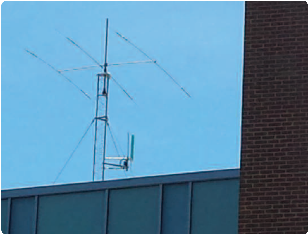
Figure 4: View of the Kingsbury Antenna Tower from the North
