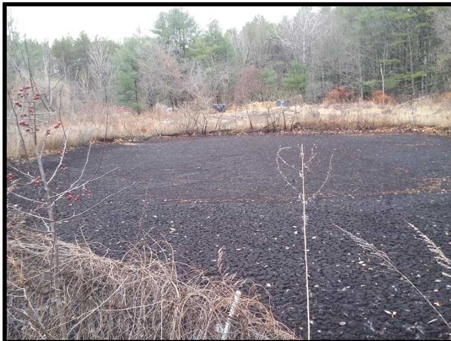
Figure 1: WTR Lagoon at the Durham, NH Drinking Water Treatment Plant
