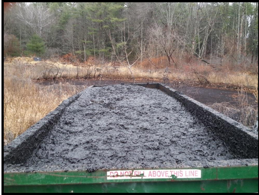
Figure 2: WTR loaded directly into 30 cubic yard dumpster in the fall.
