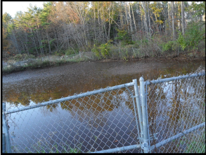
Figure 9. WTR Lagoon at the Durham Drinking Water Treatment Plant.
