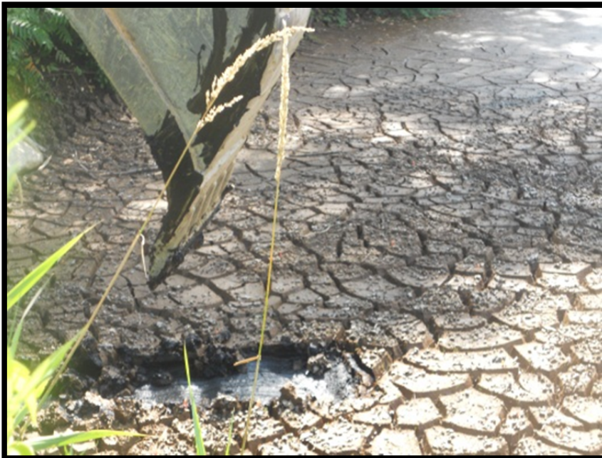
Figure 10. Far side of WTR lagoon at Durham Drinking Water Treatment Plant.
