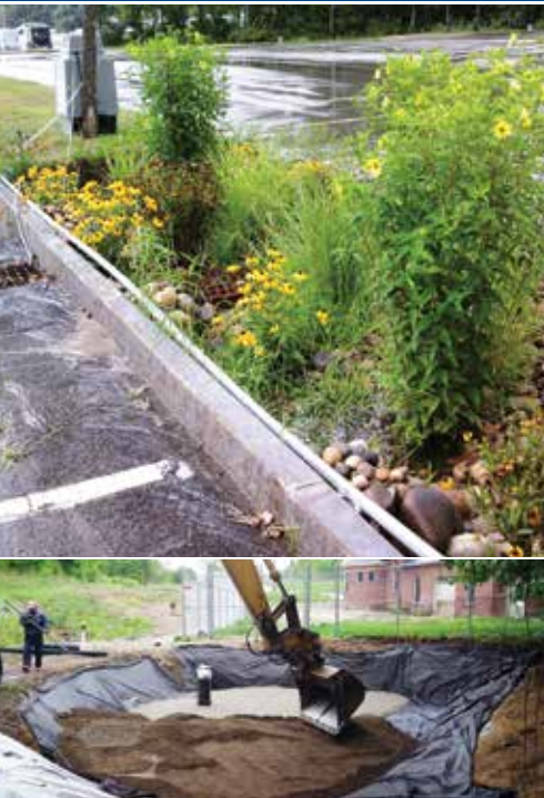
Soil media composition largely determines a bioretention system's ability to treat water quality.
