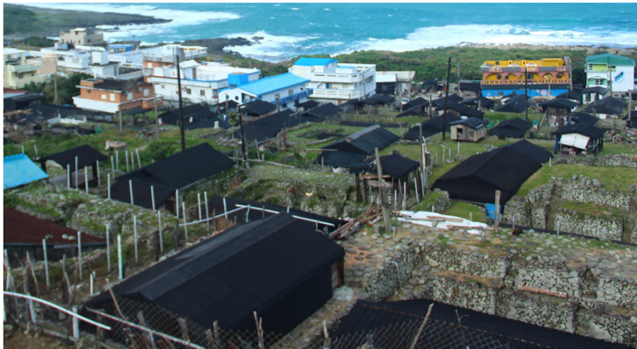
Fig. 4. Traditional houses (those with black roofs) at Lanyu (a small island off the east coast of Taiwan), constructed mostly below ground with a drainage system to resist typhoon effects as well as mitigate summer heat.
