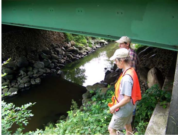
Figure 2. Assessing Crossing at Route 33 Bridge, Greenland (D. Bechtel TNC)
