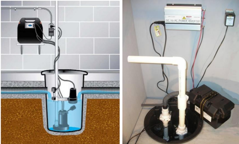
Figure 10- Battery Backup [33]
