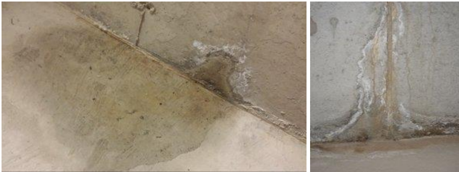
Figure 12- Foundation Crack [36]
