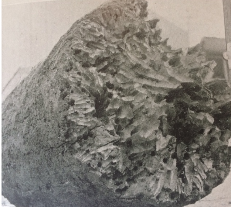
Figure 10: Hollowed Wood. From the outside, infested piles and planks appeared unharmed. But when opened, they could be completely perforated. Credit: The San Francisco Marine Piling Committee of the American Wood-Preservers' Association, Inc. [ First ] Report on the San Francisco Bay Marine Piling Survey , plate 13. Used with permission of the American Wood-Preservers Association.
