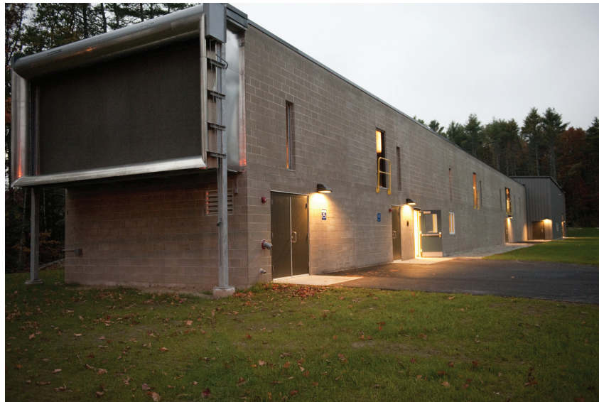
FIGURE 2.6: FPF wind tunnel, air flow enters the test section through the inlet at the front and discharges into the atmosphere at the rear.
