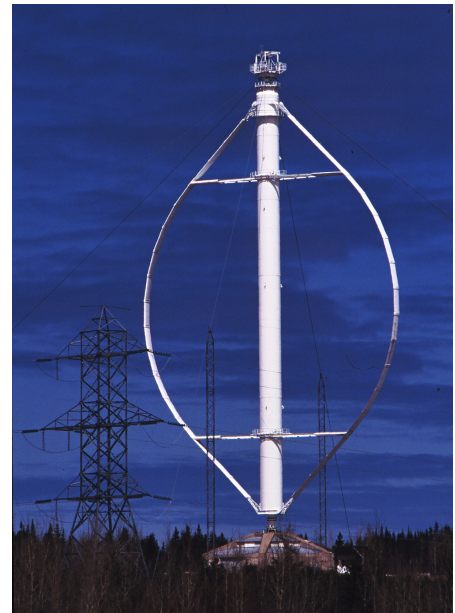
(b) Lavalin Eole 64 m diameter VAWT. Photo by Paul Gipe. All rights reserved.
