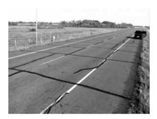
Figure 2.8: Thermal cracks in asphalt pavement (Dongré and D'Angelo, 2003)
