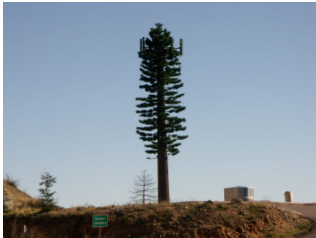
Figure 1.1: An antenna disguised as a tree to reduce its obtrusiveness to the environment [1].
