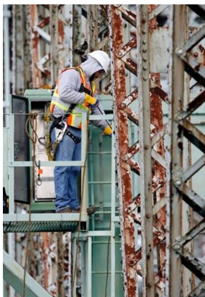
Figure 27 – Degradation of the original Memorial Bridge truss system (Jim Cole, 2010)
