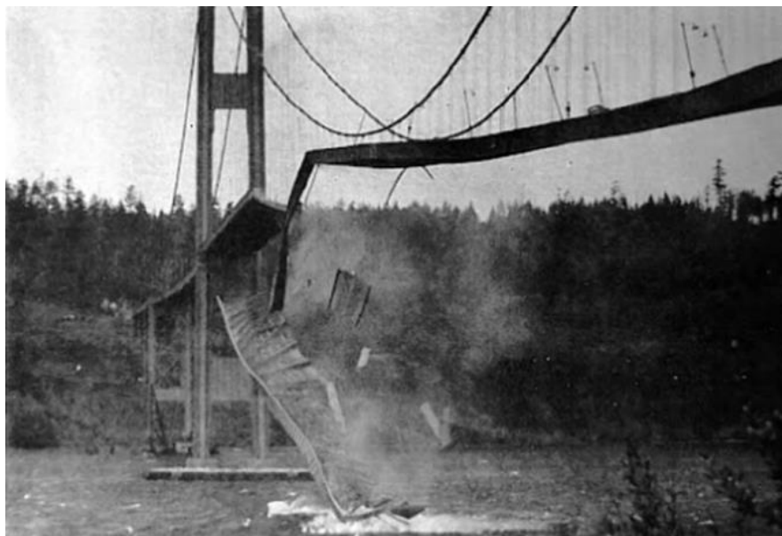
Figure 5 - Collapse of the Tacoma Narrows Bridge
