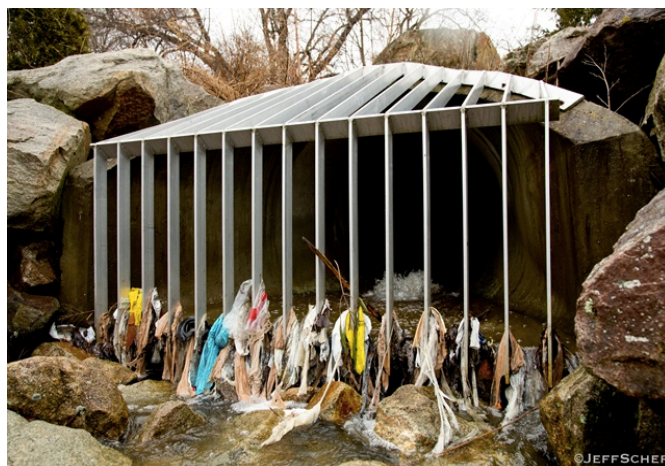
Figure 11: Plastic bag litter in stormdrains and infrastructure impairment (Portland, n.d.).
