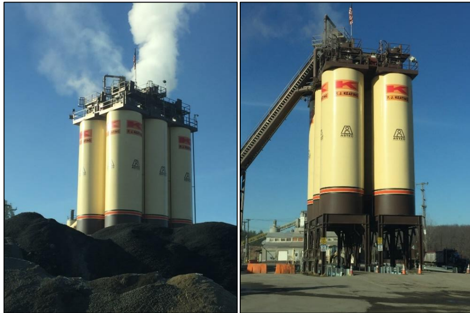
Figure 3: Example of Storage Silos
