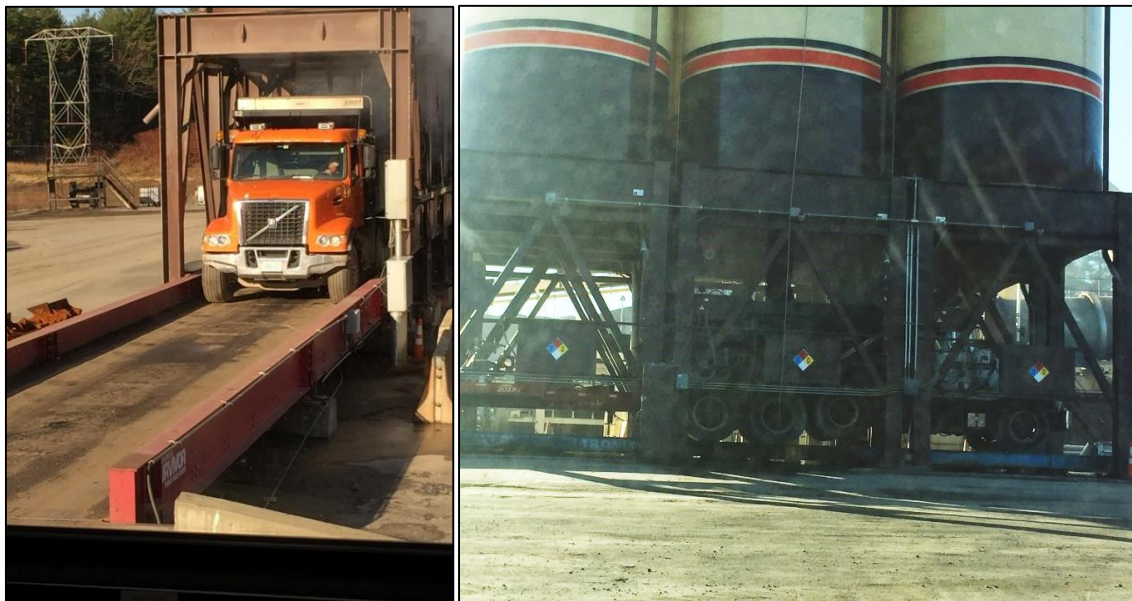
Figure 4: Example of Material Being Discharged from Silos to Trucks
