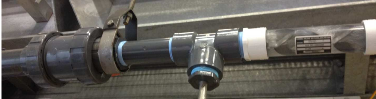
Figure 3.9 Komax static inline mixer placed in horizontal pipe
