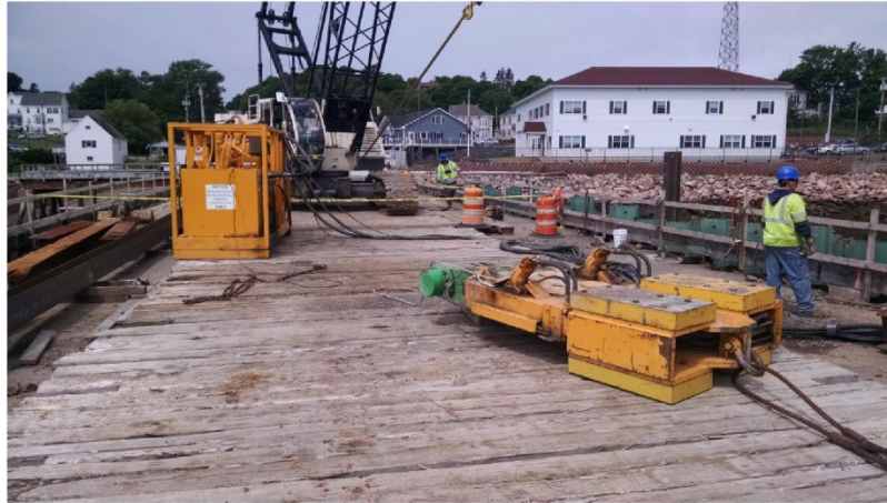
Figure 5 - H&M 3400 Hammer and Power Pack
