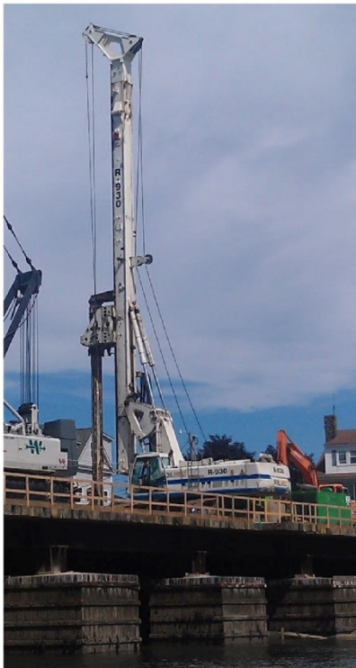
Figure 2 - Soilmec R-930 On North Trestle
