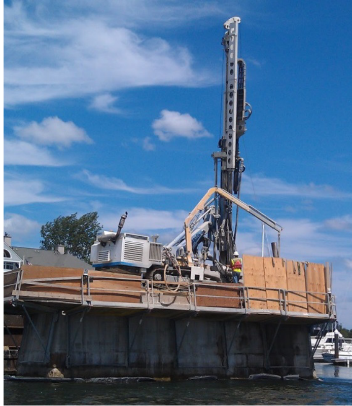
Figure 10 - PSM - 1350 Hydraulic Drill Rig Installing Micropiles on Pier 4
