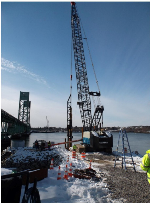
Figure 6 - Bermingham B64 Diesel Hammer
