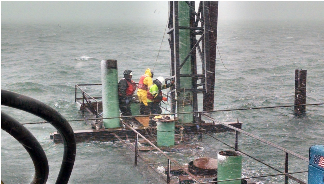
Figure 53 - Driving Battered Piles at High Tide
