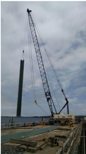
Figure 4 - Handling 65 foot Sheet Piles
