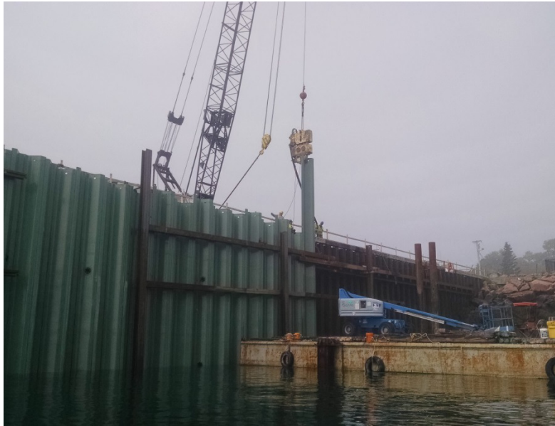
Figure 38 - Driving PZC-18 Sheet Piles with an H&M 3400 Hammer
