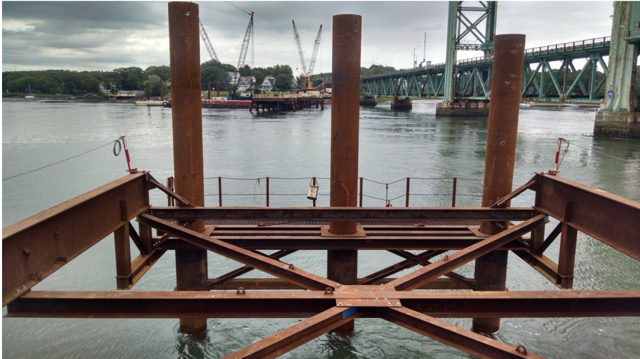
Figure 27 - Piles in Cantilevered Template After Driving
