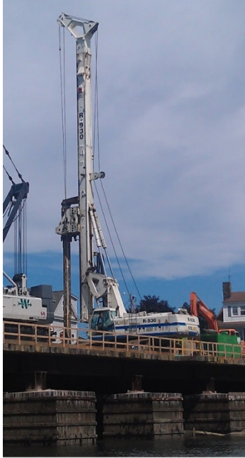
Figure 11 - Soilmec SR-930 Installing a 36" Diameter Drilled Shaft
