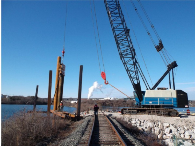
Figure 5 - APE Model 200 Vibratory Hammer
