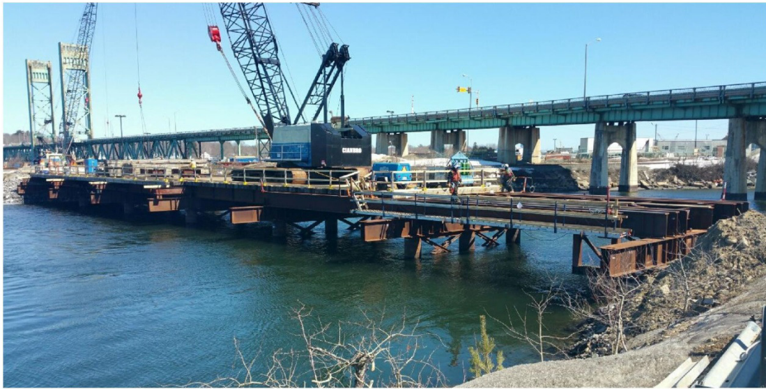
Figure 2 - Cutt's Cove Trestle Nearing Completion as Seen From Market St.
