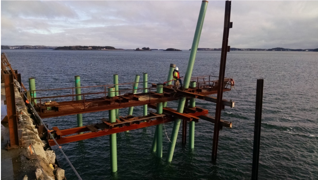
Figure 52 - Battered Piles in Template at Low Tide
