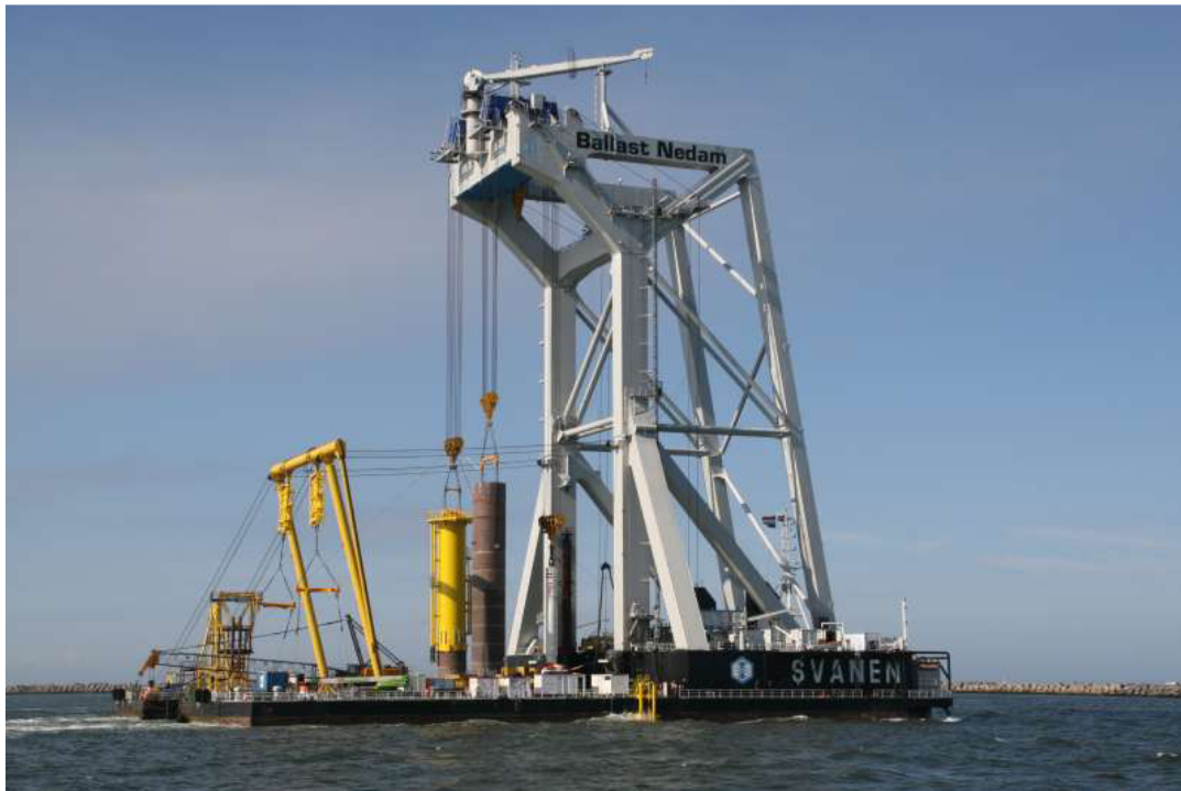
Figure 1 – HLV (Heavy Lift Vessel) “Svanen” Installing Monopiles in the North Sea
