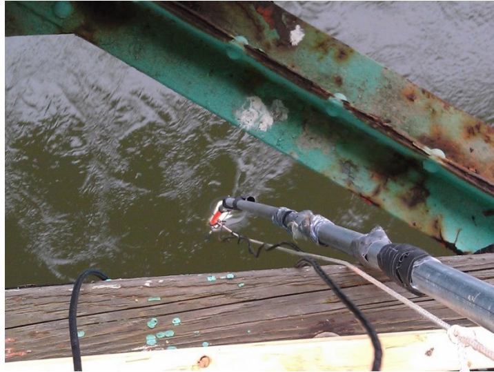
Figure 14 - Deployment of Hydrophone Through EMT Conduit Below the SML Bridge
