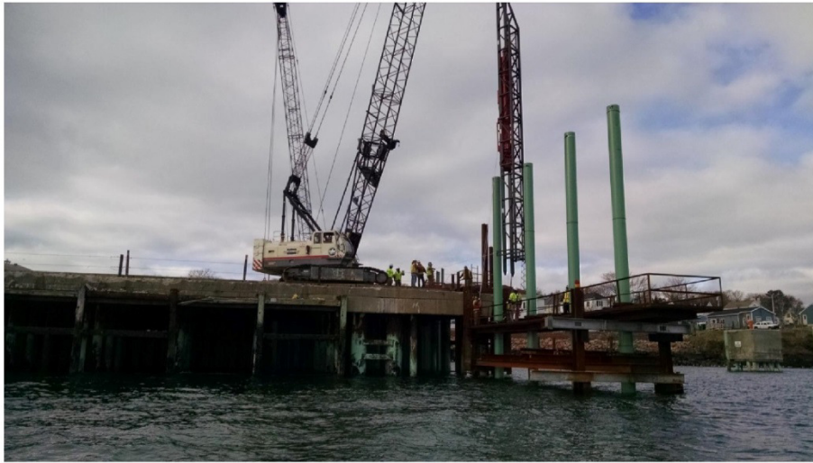
Figure 5 – Pileco D30-32 Hammer In Use on Bent 1
