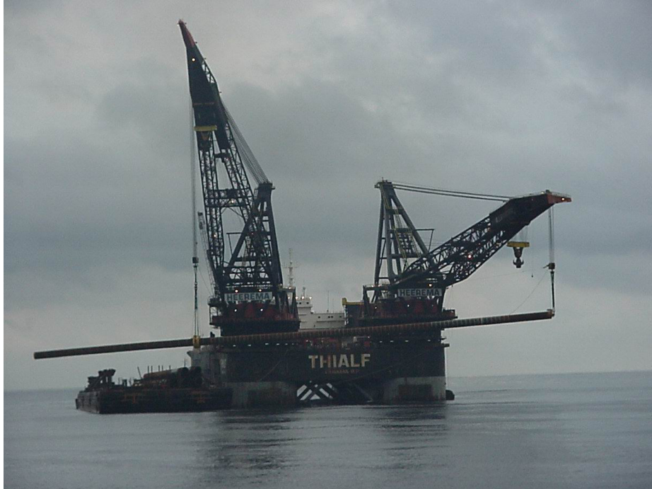
Figure 2 –“Thialf” World’s Largest Crane Vessel Handling 800’ Piles for an Offshore Platform Jacket
