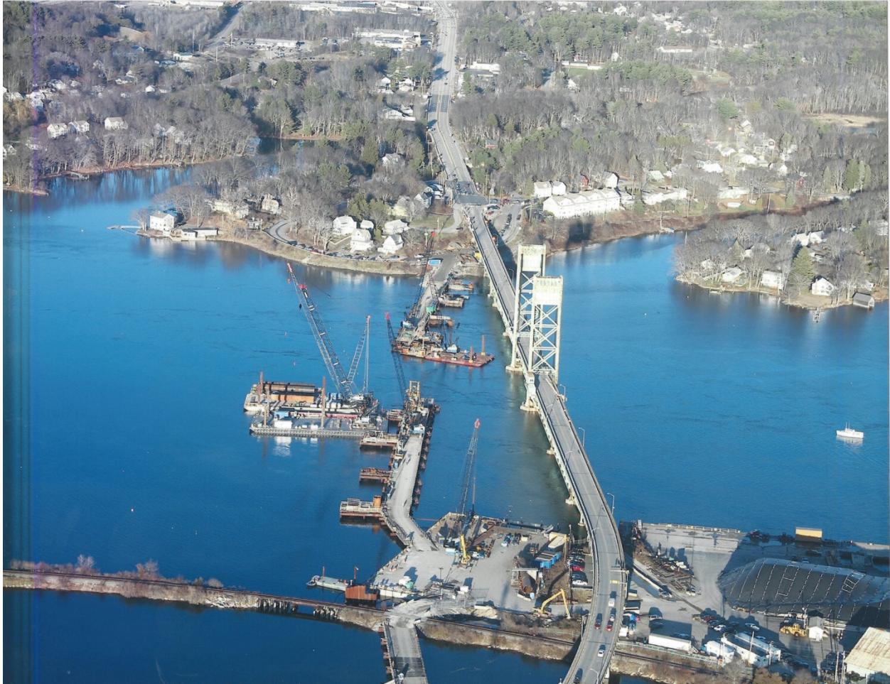
Figure 22 - Overview of Completed Temporary Crane Trestles
