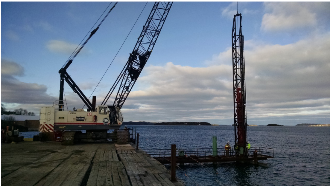
Figure 50 - Driving 20" Pipe Piles with a Pileco D12 Diesel Impact Hammer
