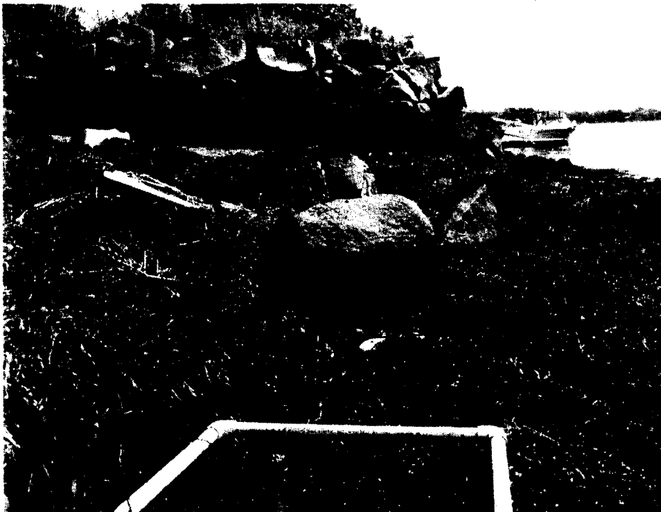
Figure 32 Cedar Point boat launch A) facing south B) facing north with boat launch and retaining wall.
