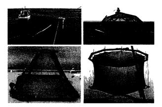
Figure 7.15: Cage systems deployed at the site include the SeaStation<sup>™</sup> (top left), Aquapod<sup>™</sup> (top right), OCAT (lower left), and the JPS prototype (lower right).
