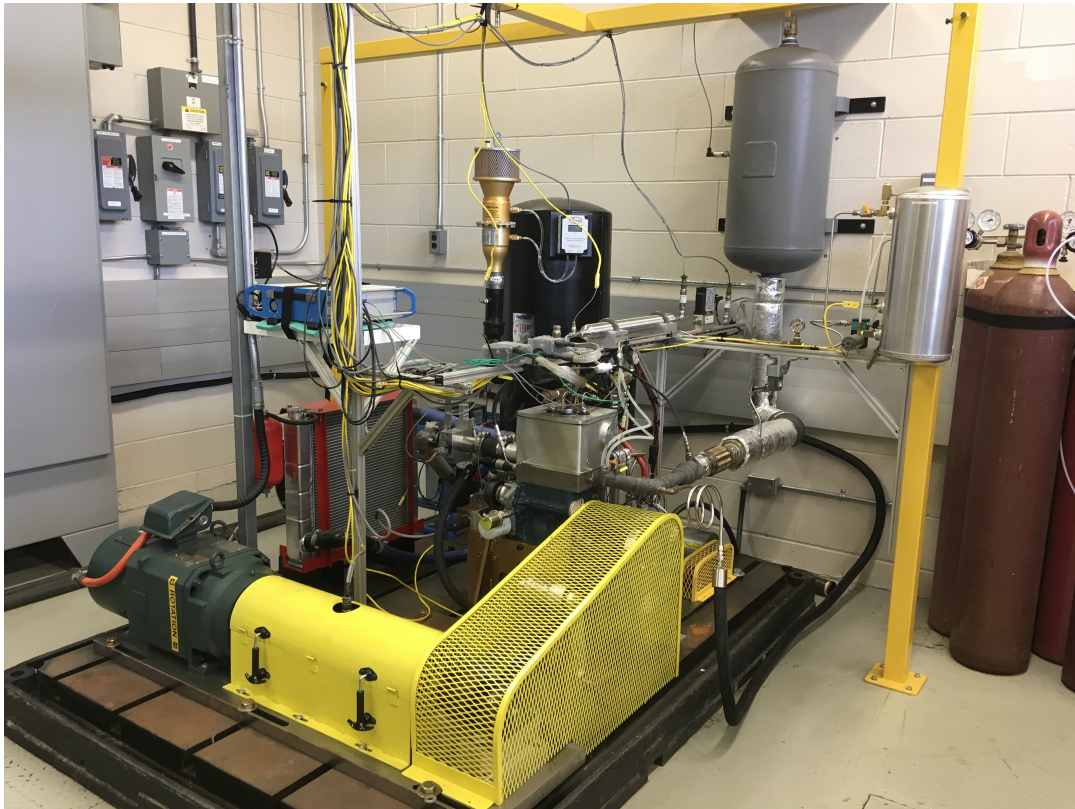
Figure 2.5: Engine Dynamometer Set-Up
