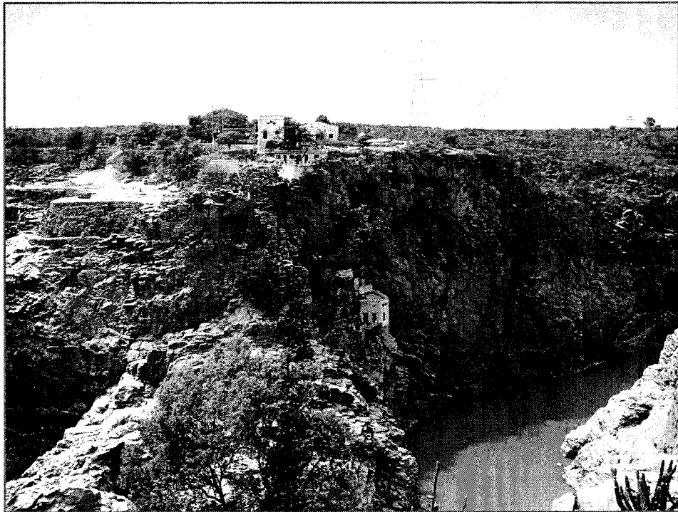
Figure 1.1. Delmiro Gouveia Hydropower Station Source: Lucigleide Nascimento 2002
