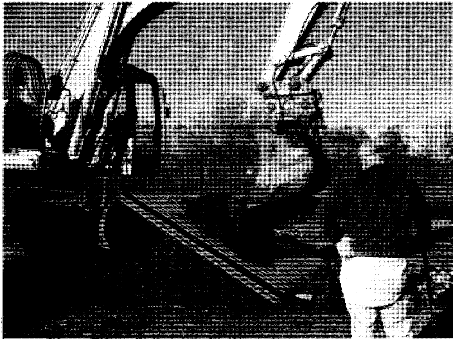
Photo 4.2 Screening the sediment to remove rocks and other large objects.
