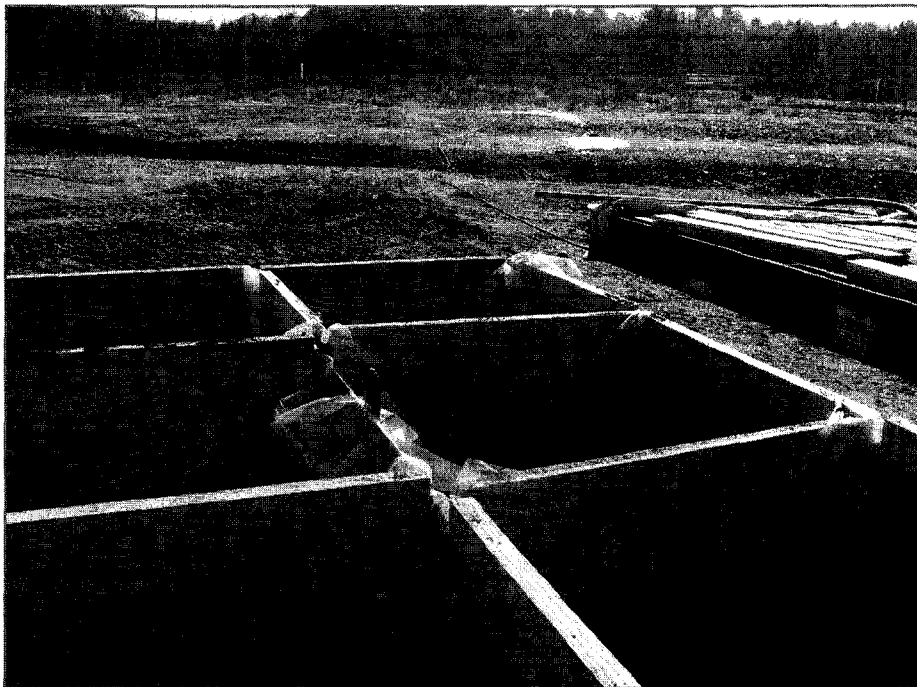
Photo 4.6 Plastic liners installed in the test cell module.
