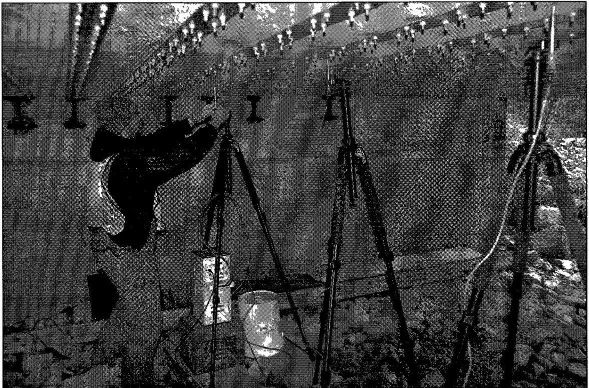
Figure 12 – Installation of LVDT equipment underneath the bridge in Gilford, NH, post-renovation.
