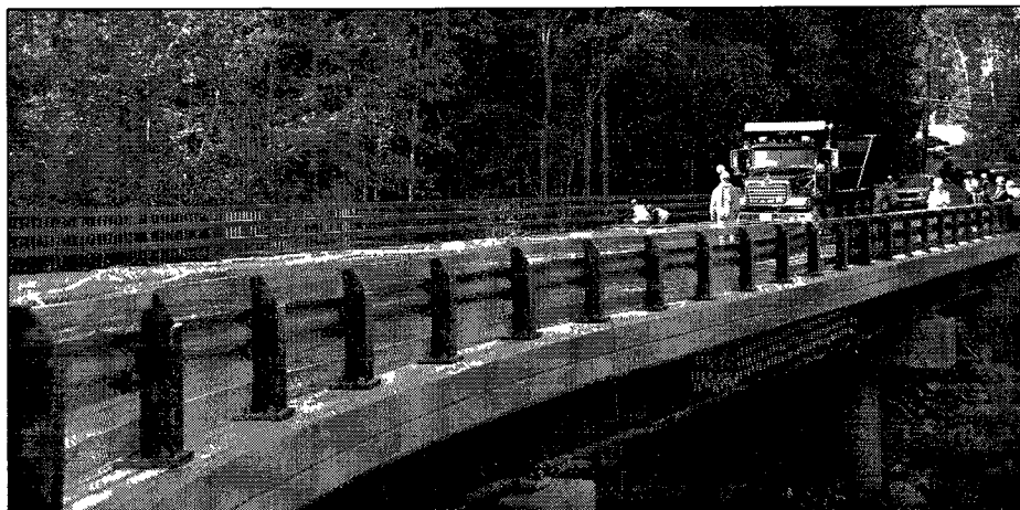
Figure 11 – The newly constructed Vernon Avenue Bridge.
