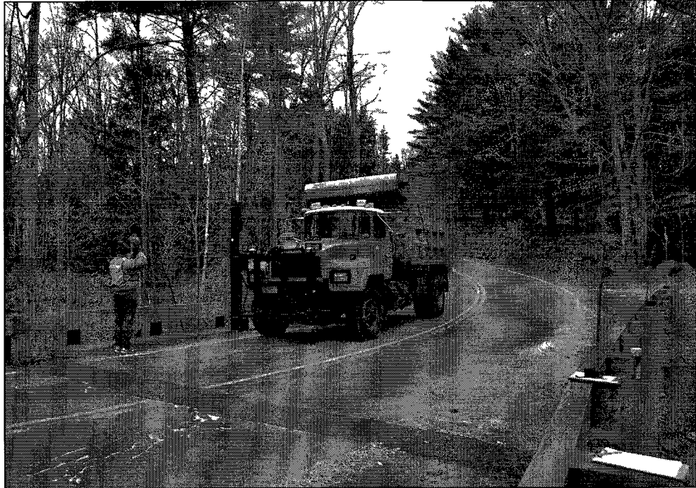
Figure 15 - View of the top of the bridge and load truck in Gilford, New Hampshire.
