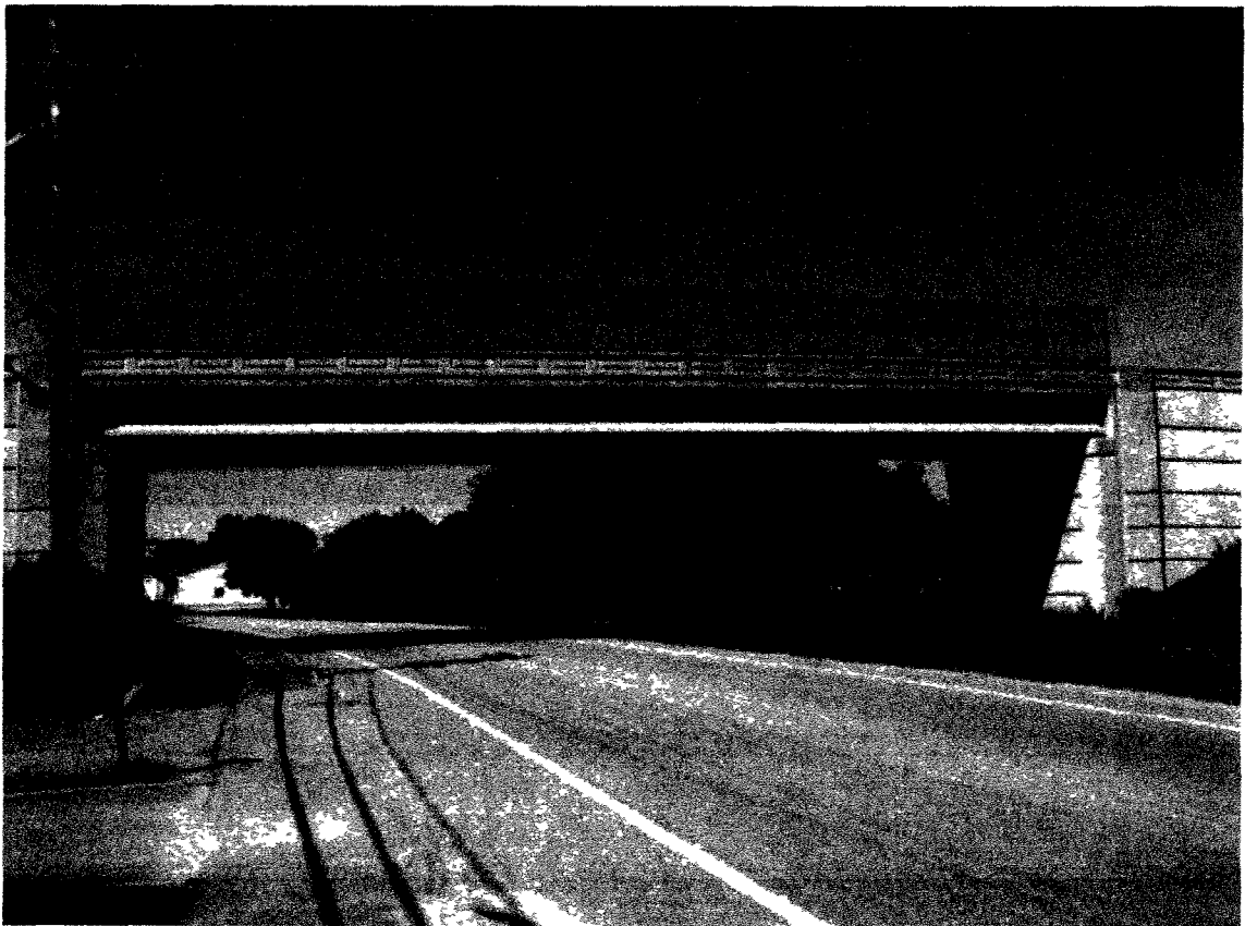
Figure 31: Rollins Road Bridge
