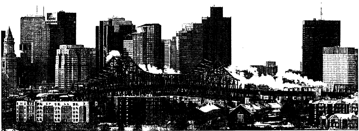
Figure 4. Boston's Tobin Memorial Bridge is instrumented for SHM and proactive maintenance
