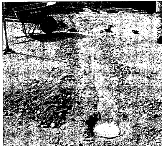
Figure 37. Pressure cells installed in subgrade prior to paving
