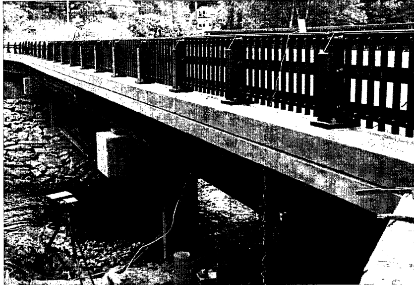
Figure 96. South Span Camera Setup Location
