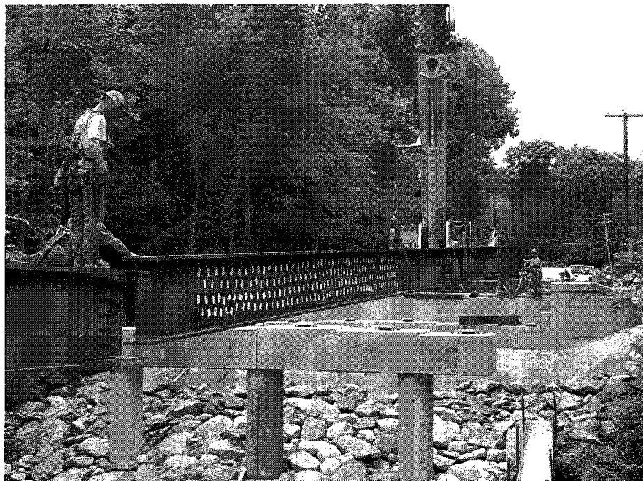
Figure 5-2: Girder 1 being installation with speckle pattern in place
