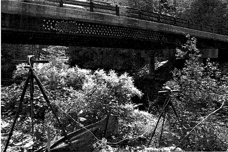
Figure 5-7: Middle span DIC setup
