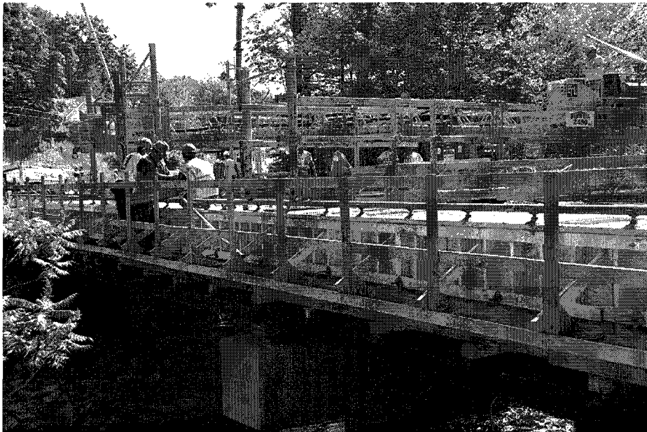
Figure 5-5: Concrete deck pour and heavy equipment operation
