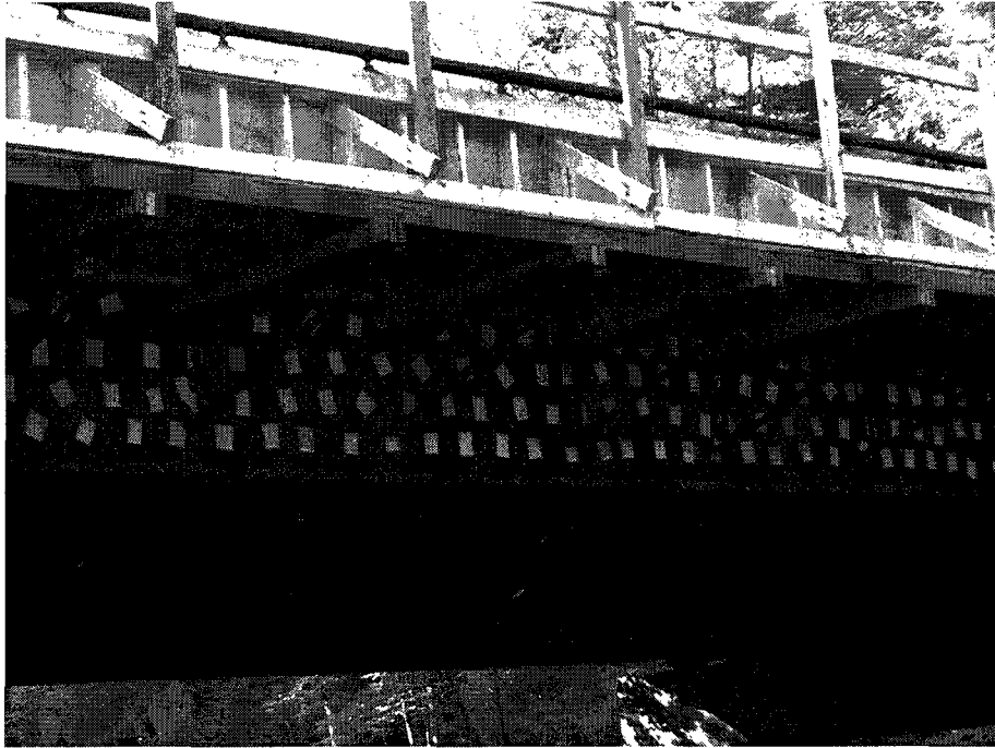
Figure 5-3: Vernon Avenue Bridge speckle pattern with obstructions
