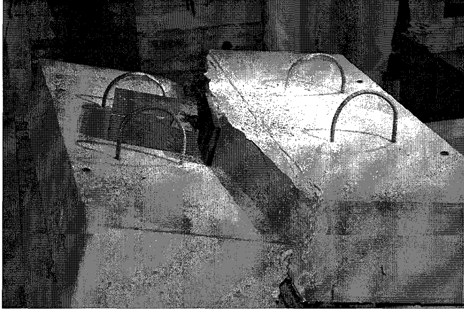
Figure 4-8: Slab after failure
