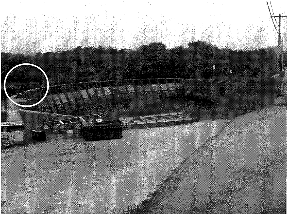
Figure 4-22: Pond Bridge Road Bridge DIC test setup
