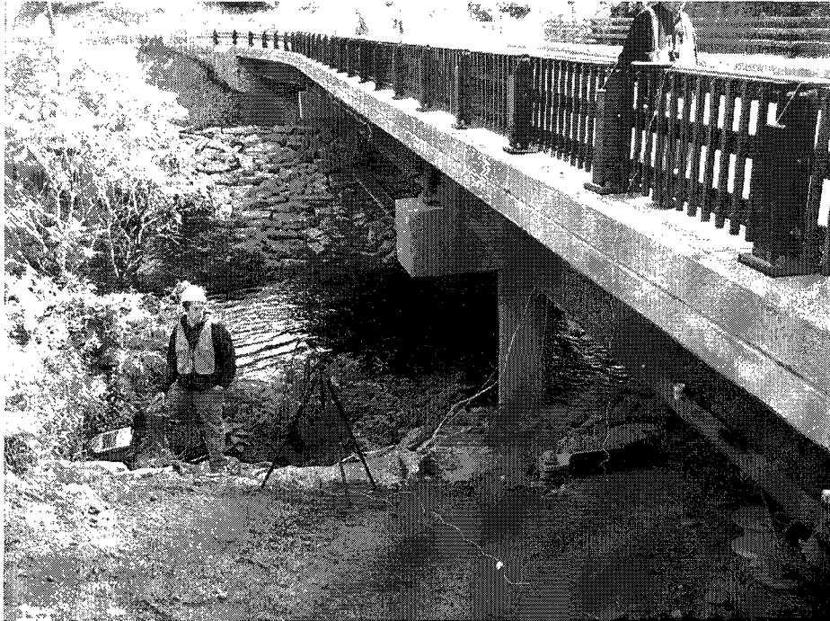
Figure 5-10: DIC setup at south span
