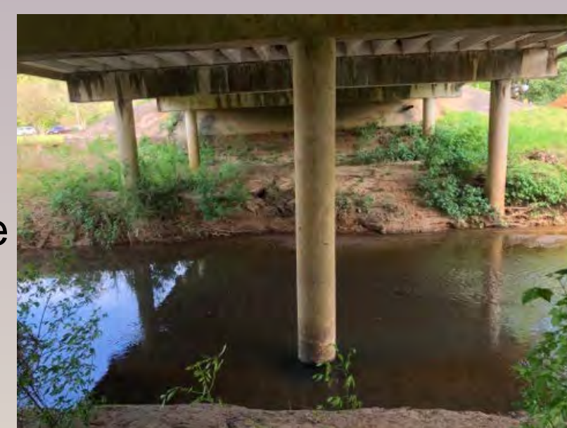
College Street Bridge
