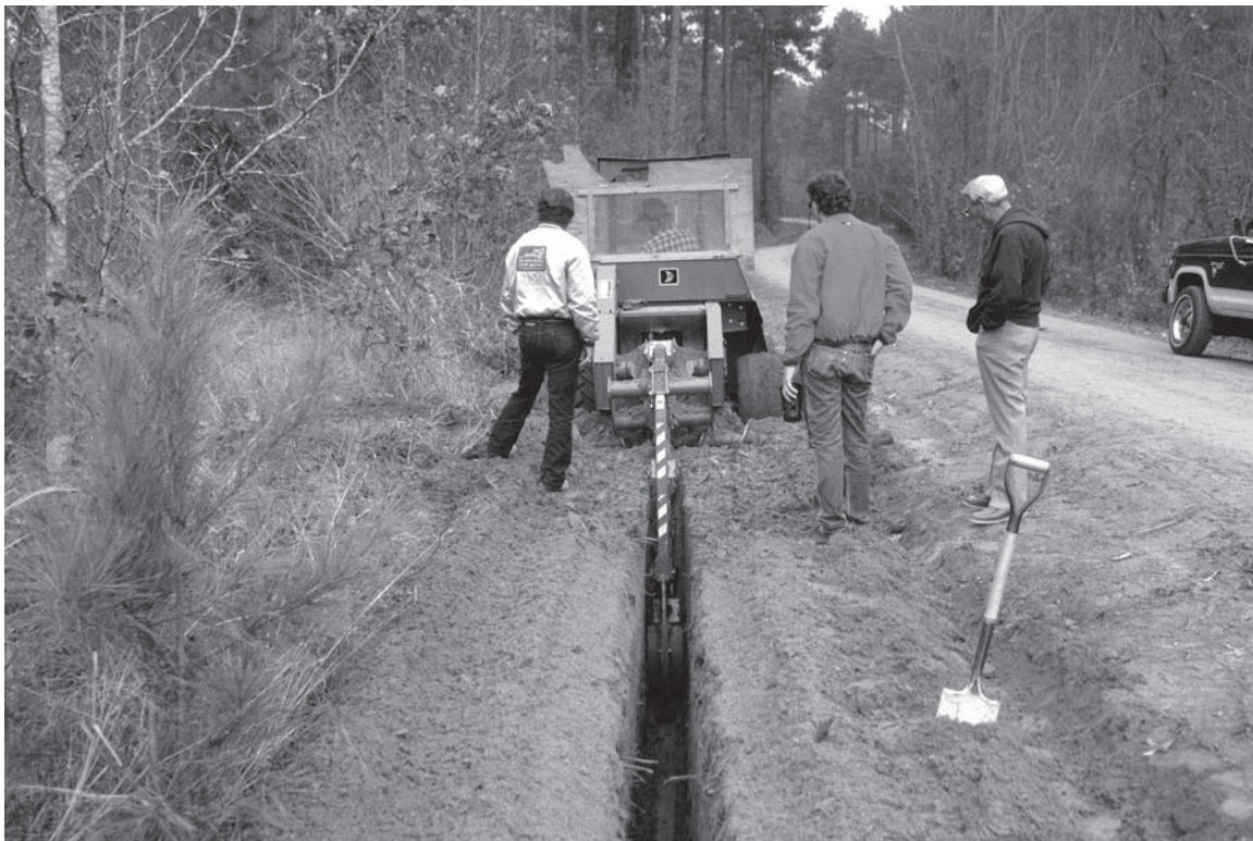
Figure 3. Digging of the pipeline trench to the gas well.
