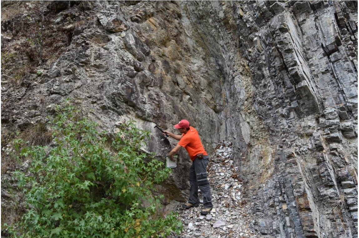
Figure 2.10. Contact between Lower Novaculite breccia subdivision (left) and Middle Chert and Shale Member (right) at the northern section of the Caddo Gap road cut. North is to the left.
