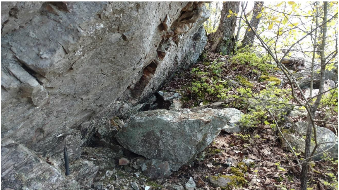
Figure 4.17. Same fault surface at Stop 500, about 300 feet away. Footwall rocks were densely fractured to brecciated. Faint fault grooves (?) and conflicting chatter marks indicated both oblique left-lateral normal and oblique right-lateral reverse sense of slip. View is looking west, hammer for scale.
