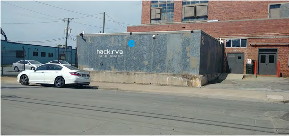
Figure 18: Street level view of Parklet Site 1
