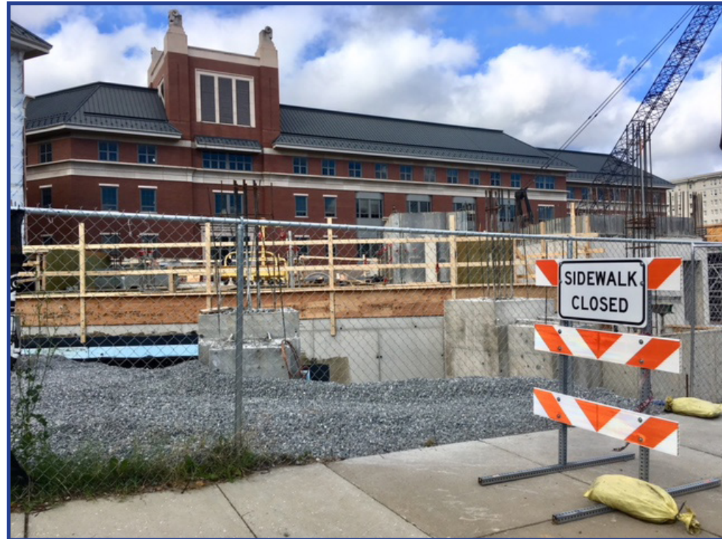
Figure 19: Location of Former Green Lawn next to Snead Hall
