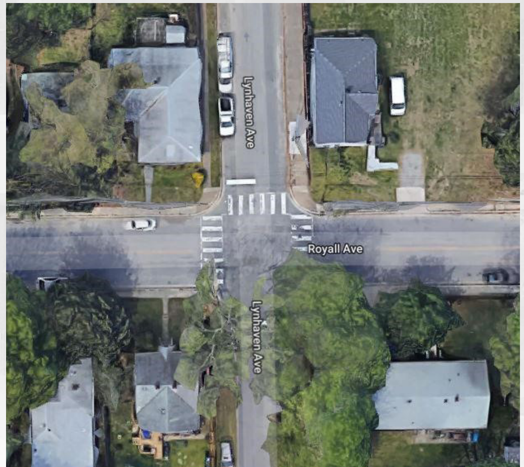
Figure 17: Birds eye view of intersection leading to elementary school and community center
