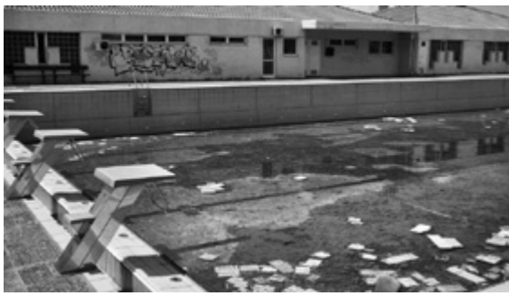
Fig. 7 In the former training pool for the 2004 Olympic swimmers, trash floats on four inches of stagnant water.
