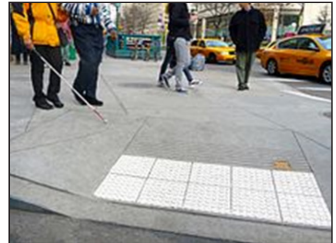
Figure 53: ADA Wheelchair Ramp Crosswalk
