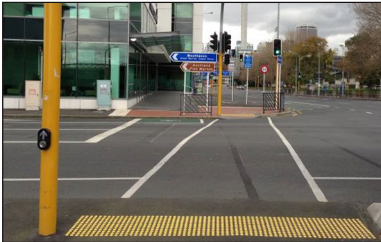
Figure 52: ADA Compliant Crosswalk for Wide Streets
