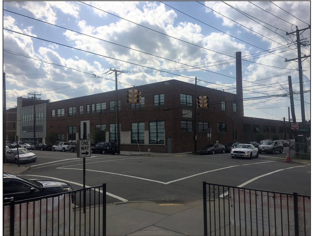
Figure 67: Before - Roseneath Rd. and W Clay St.
