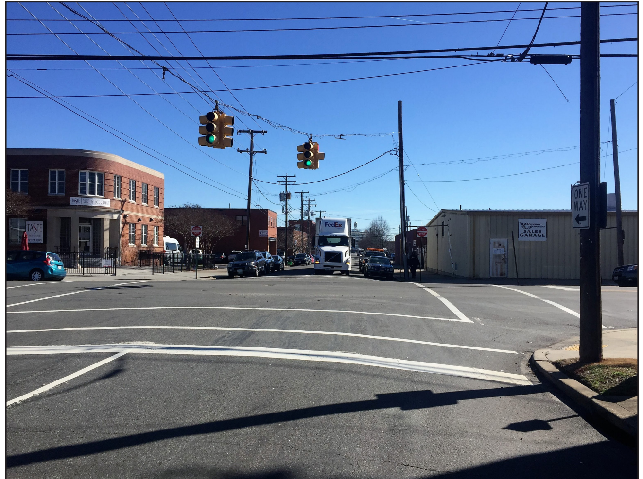
Figure 73: Before - W Clay St. Ramp
