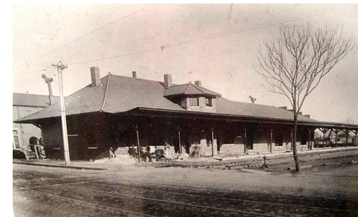
HULL STREET STATION | SOURCE: RICHMONDRAILROADMUSEUM.ORG
