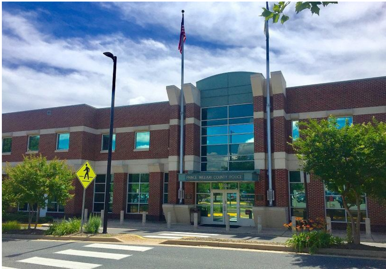
Figure 13 Eastern District Police Station, Main Entrance
