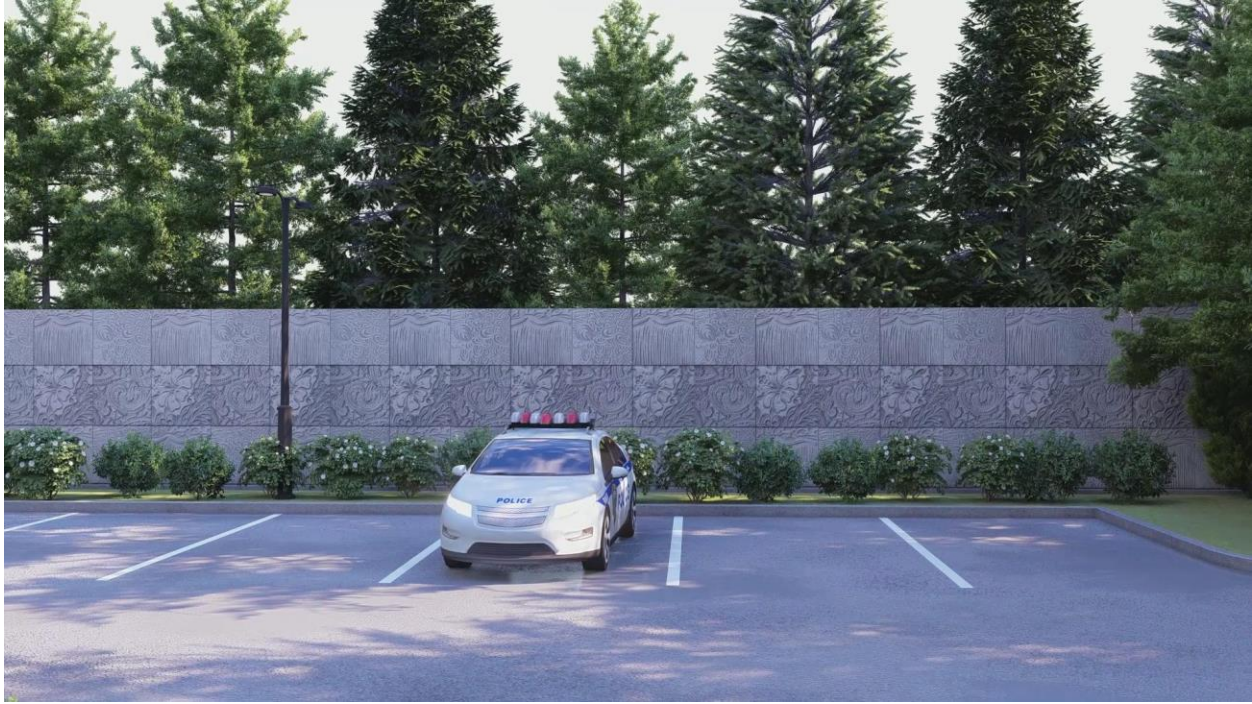
Figure 41 The Fourth District Police Station Rear Wall
