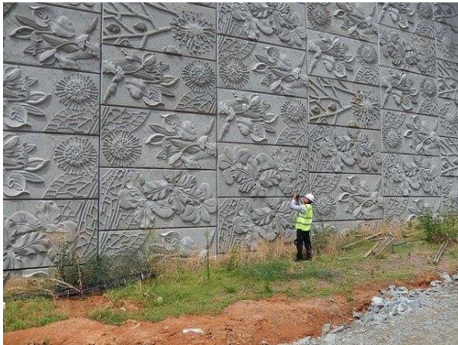
Figure 40 Concrete Wall That Incorporate Artwork
