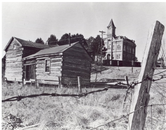
Figure 1. The Ficklin-Imboden log house is depicted in this historic photograph of the log structure (left) and the Lawrence County Courthouse (right) taken in ca. 1940 (photo courtesy of K. Watts). Both structures have been stabilized and restored as part of Powhatan Historic State Park
