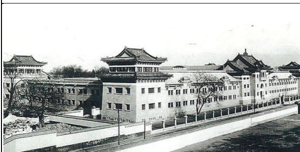
Figure 1.13. The College of Clergy of Peking Fu Jen Catholic University in 1937, designed by Dom Adalbert Gresnigt. Photographed from Qing-Zhen Mao, “Regarding the 90th Anniversary of Fu Jen Catholic University,” The Observer, accessed March 31, 2019, https://www.observer-taipei.com/article.php?id=1188 .
