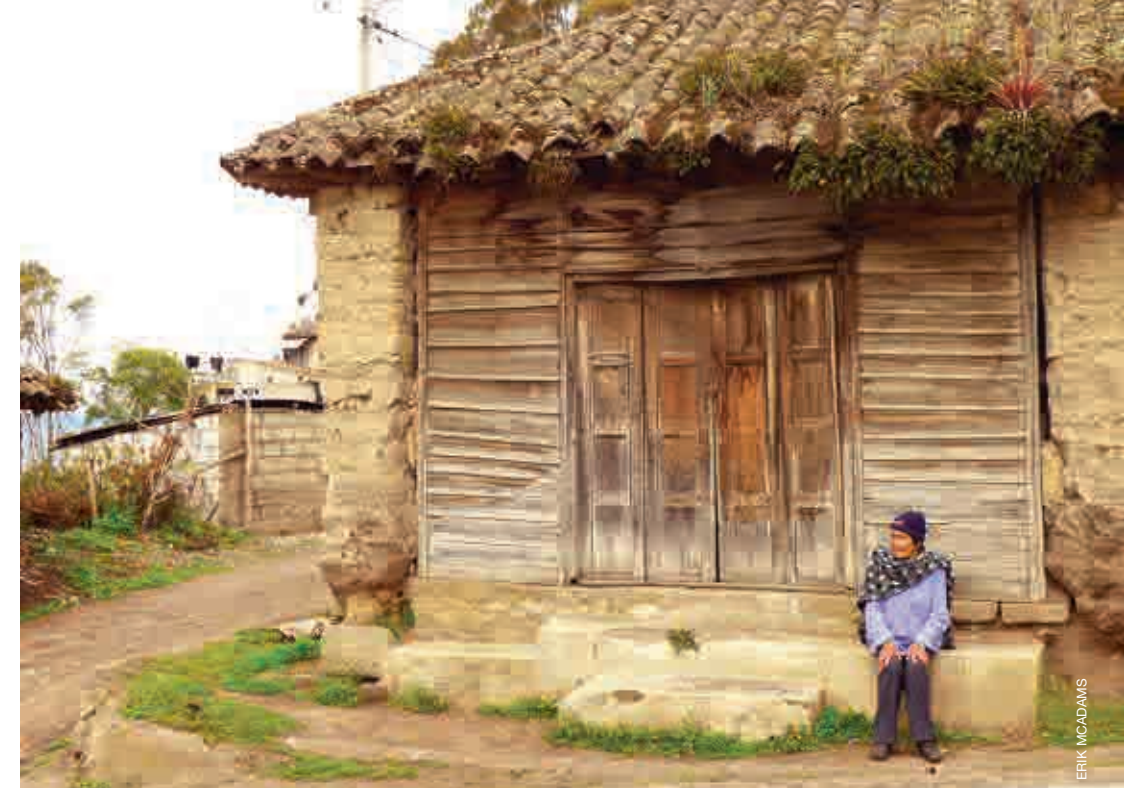
Strong point: One of the few rural homes to survive the devastating 1949 earthquake, this adobe house near Ambato, Ecuador, has meter-thick walls reinforced with skinny strands of bamboo.
