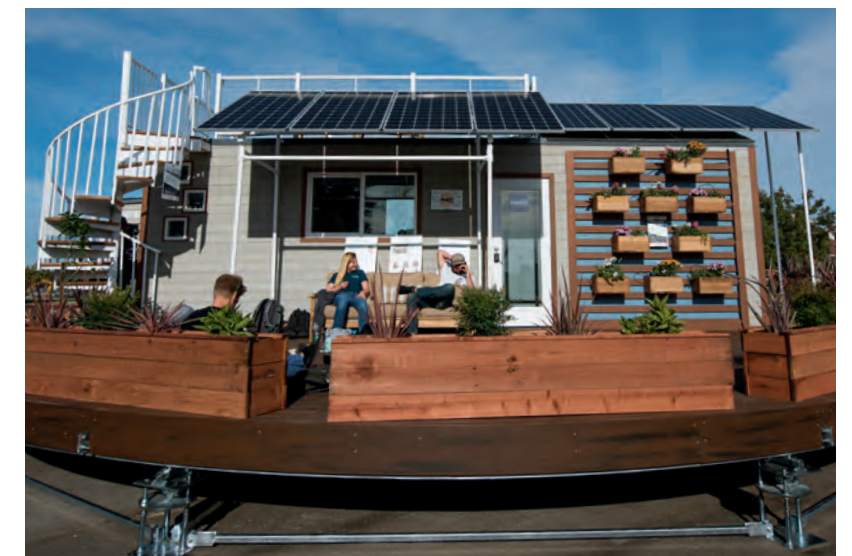
One good turn: the house and the base that lets SCU’s rEvolv House spin
