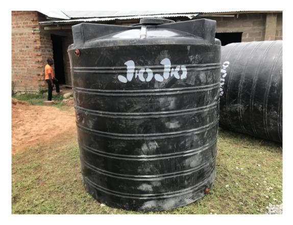
Figure 14: 10,000 L tank with brown <sup>3</sup>/<sub>4</sub>" gaskets installed at the top and bottom of the tank.
