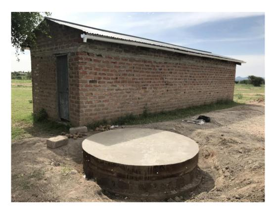
Figure 13: Finished non-potable tank foundation in the process of curing. During the time that the team was on the construction site, three tank foundations were constructed: two (2) potable-use tank foundations and one (1) non-potable-use tank foundation.
