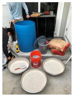
Figure 8: Assembly of slow sand filter.
