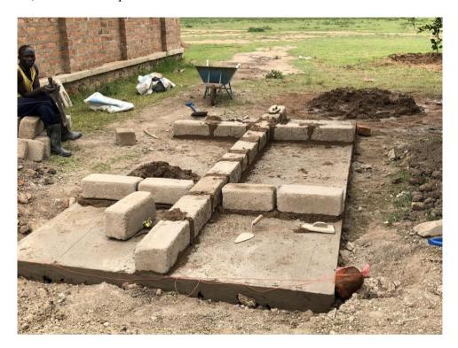
Figure 12: First layer of brick for the cross foundation.
