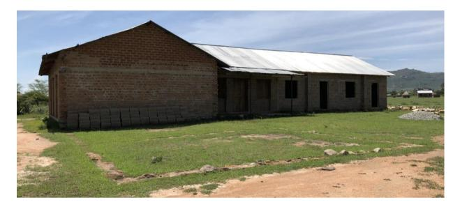
Figure 15: Construction progress of Buturi community center as of March 27, 2018. Dirt outline indicates foundation boundary and area of future construction.
