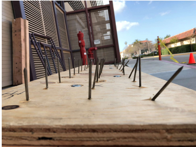
Figure 7: Nail connection to top earthbag layer.
