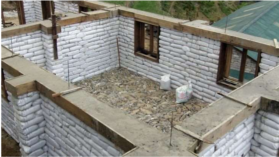
Figure 3: Earthbag home built with concrete bond beam.
