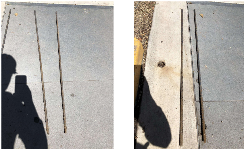
Figure 26 (L) and 27 (R): Rebar used in Wall 2.
