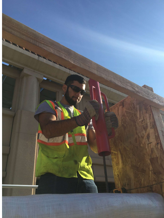
Figure 13: Driving sharpened rebar into wall.
