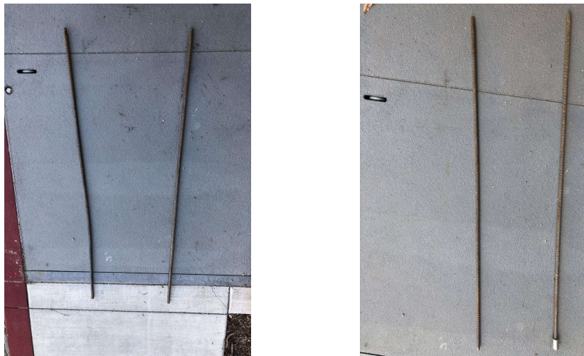
Figure 24 (L) and 25 (R): Rebar used in Wall 1.
