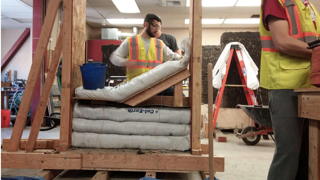
Figure 6: Construction practice used to build both wall specimens.
