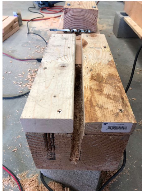
Figure 8: Guide channel at ends of bond beam.
