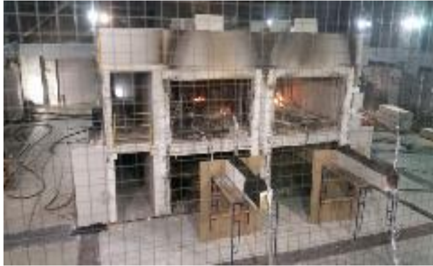
Figure 6: AWC test building for CLT fire resistance research. Source: American Wood Council, 2017.
