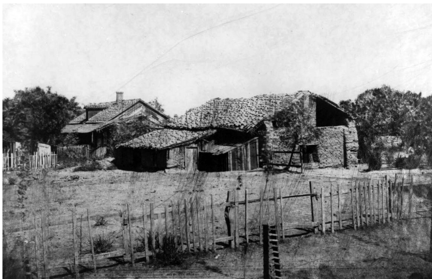
Figure 5. Remnants of adobe neophyte barracks, ca. 1868. The structure in the background houses the Santa Clara Woman's Club. Image courtesy of Archives and Special Collections, Santa Clara University Library.
