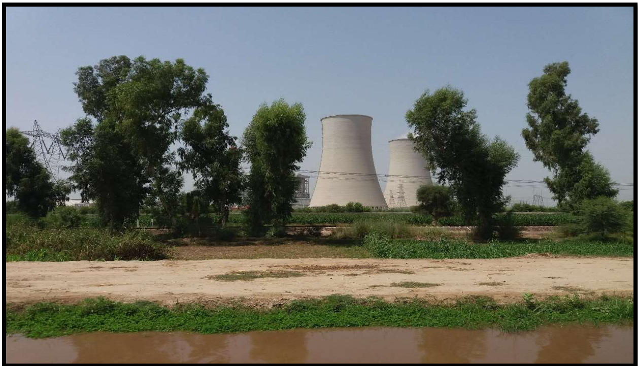
Photo 1: Sahiwal Coal Power Plant
