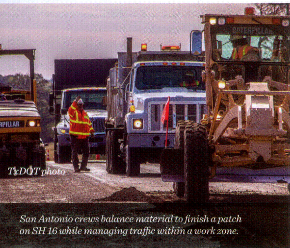
San Antonio District Transportation Maintenance Equipment Operator Brian Jasik spots for a driver while unloading cement treated black base for a patch on SH 16.
