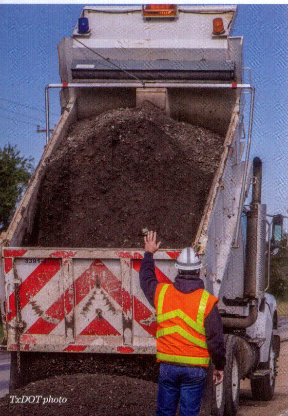
San Antonio District Transportation Maintenance Equipment Operator Brian Jasik spots for a driver while unloading cement treated black base for a patch on SH 16.
